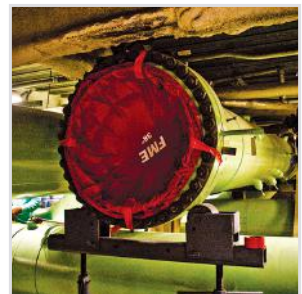
Instrumentation And Control
