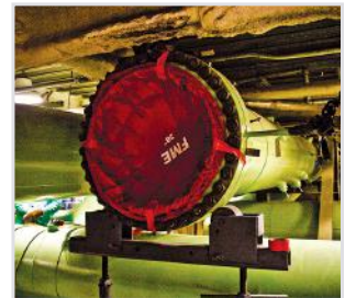
Instrumentation And Control
